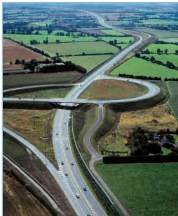
Roadstone Dublin, Ireland, supplied 260,000 tonnes of blacktop and of stonefill and 20,000 cubic metres of concrete to the Balbriggan by-pass, which comprises 13 kilometres of motorway, six kilometres of side roads, eight bridges and three interchanges. This forms part of the main route from Dublin to Belfast.
