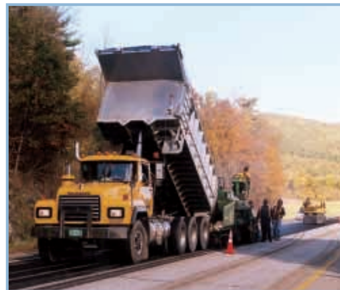
Pike industries is a leading aggregates and asphalt company in New England. This paving crew, with over 100 years of combined service, is laying hot mix asphalt on Route 4 in Rutland, Vermont.
